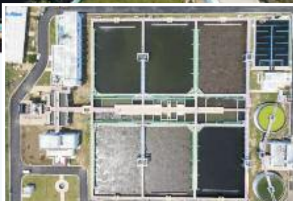
68 MLD Jagjeetpur STP made under HAM
